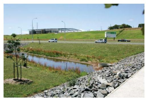
Figure 46 Storm water swales illustrates low impact storm water treatment<sup>54</sup>
